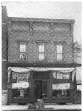
FIRST GOOD STORE IN FOREST CITY Built by J. W. Mahoney in the early '70s. Hand carved trimming by Lee Farlow, the con- tractor who erected the building.
